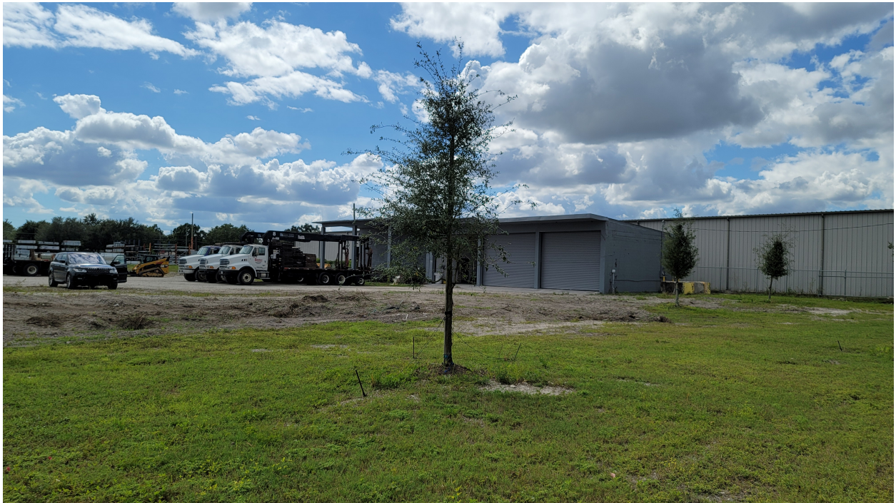
Photo 6: Looking southwest toward existing storage building where debris has been cleared.
