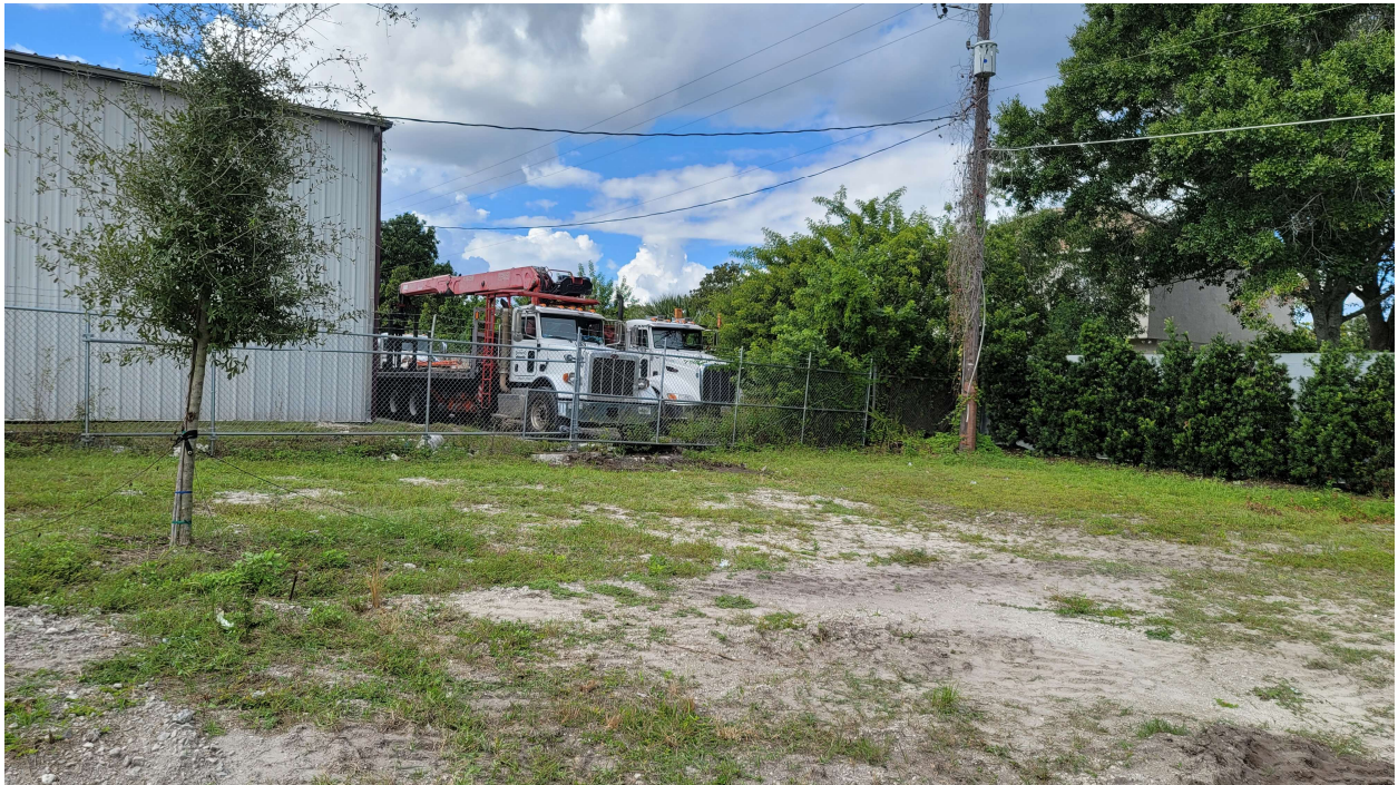
Photo 8: Looking northwest property corner at area where debris has been cleared.
