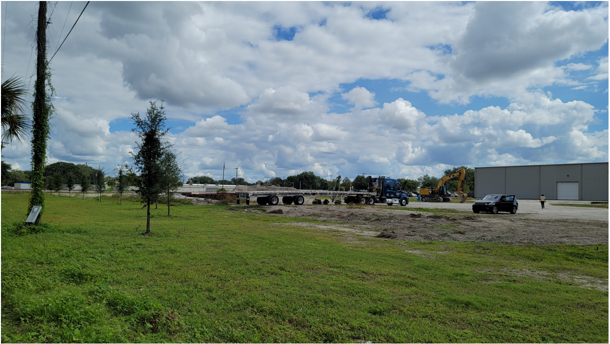
Photo 4: Looking southeast towards area where debris has been cleared.
